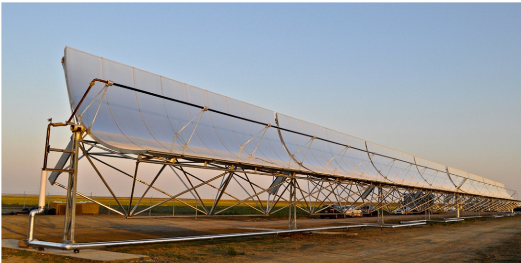
Fig. 3. The large parabolic trough solar thermal concentrator used to power the AHP–MED desalination process.
